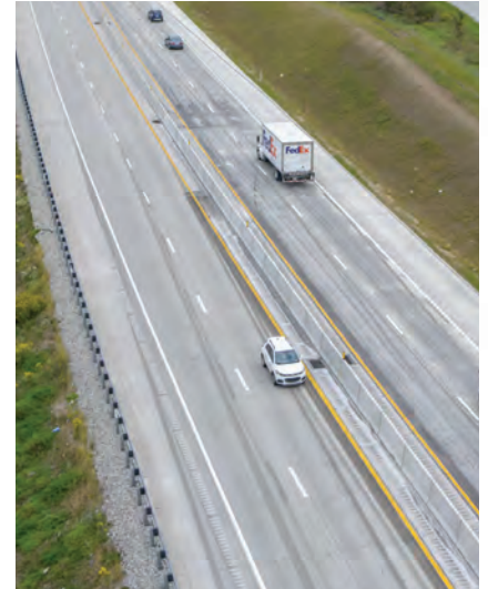
Photo from the 8th Annual Excellence in Concrete Project Award Winner Golden Triangle Construction for the SR70 Yukon & Madison Interchanges project.
