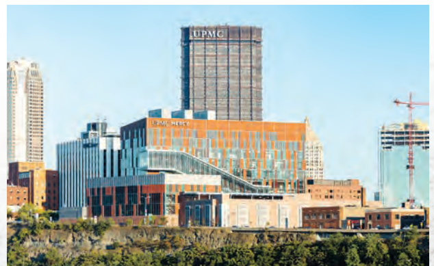
Photo from the 9th Annual Excellence in Concrete Project Award Winner Bryan Materials Group for the UPMC Vision Institute - Mercy Pavilion project.
