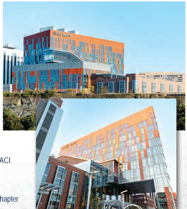
Photos from the 9th Annual Excellence in Concrete Project Award Winner Bryan Materials Group for the UPMC Vision Institute – Mercy Pavilion project.
